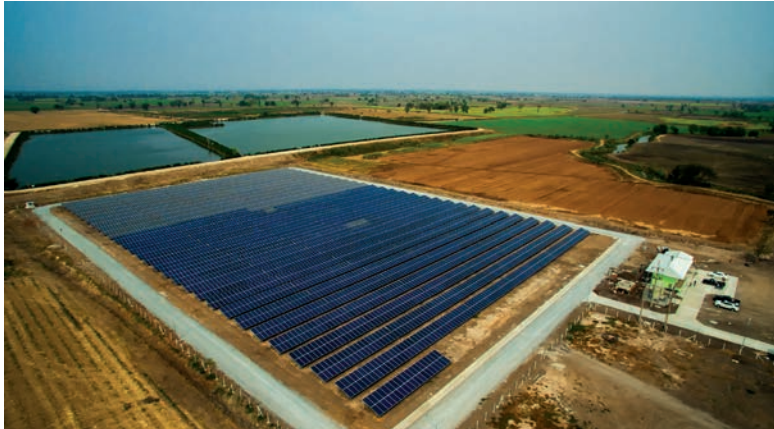
Solar farm in Dan Chang District, Suphan Buri Province
